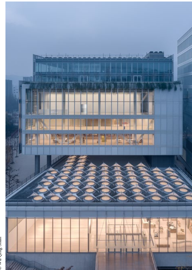
The skylight system works in conjunction with a sail shading system designed to filter the incoming daylight
