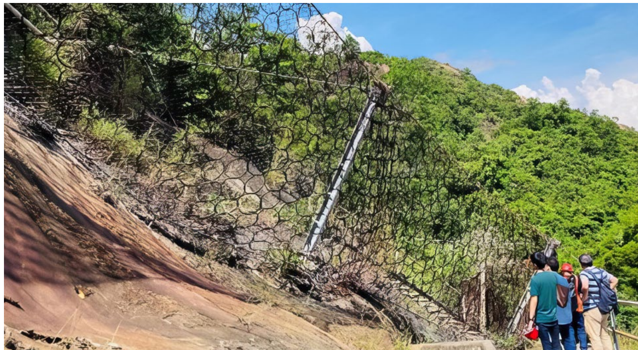
A flexible net barrier used in landslide mitigation
