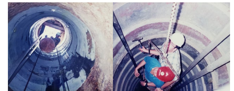
Mark inspecting hand dug caissons on Tuen Mun Road widening project in 1995
